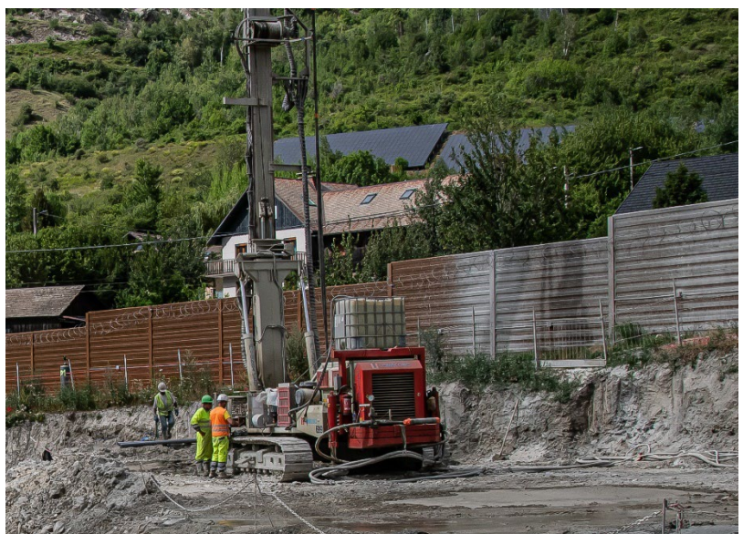
Machine de jet grouting
